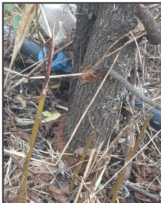
Fig. 25. Termite infestation on Tamarindus Indica (Chinch)
