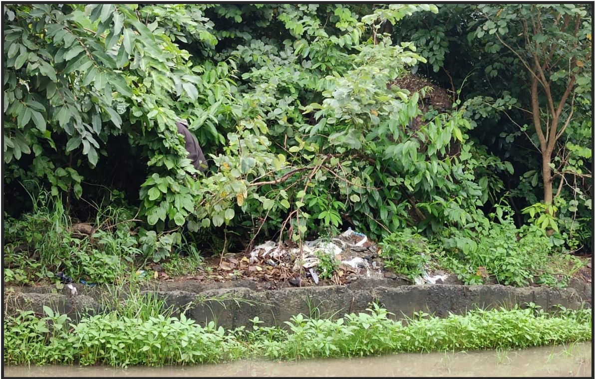
Fig. 14. Image showing the inaccessible area at the site
