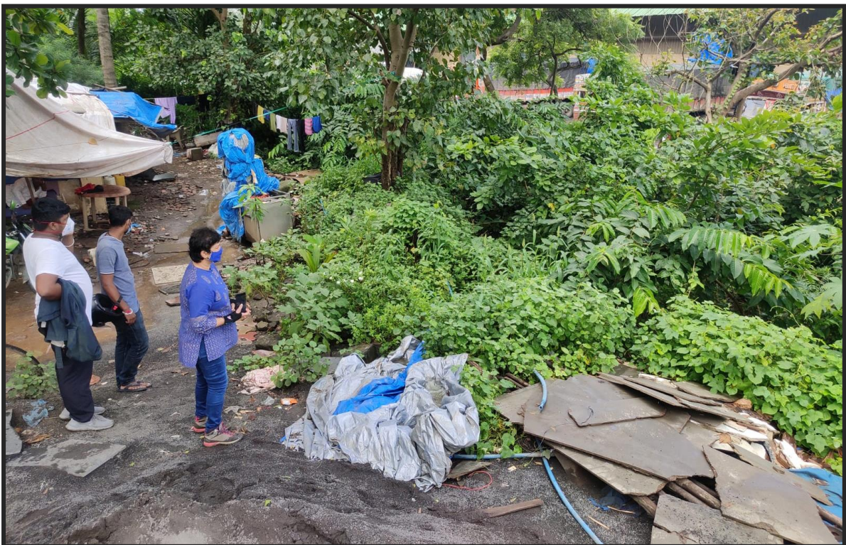
Fig. 15. Construction waste dumped in and around the site
